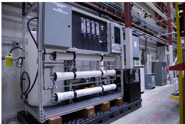
Fig 2. NREL's RO membrane evaluation experimental setup (image credit: Joe DelNero, NREL)
