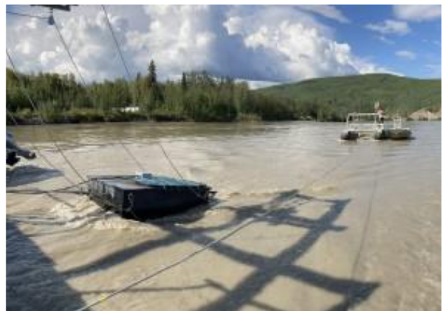
Fig. 5. BladeRunner Energy hydrokinetic turbine deployed at TRTS.
